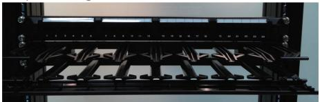
3. Insert the cords into position, plug them into the panel ports and close the hinged cover.
