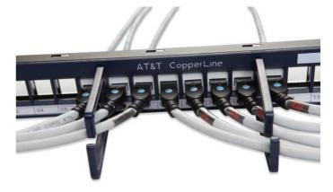
Avoid bending, kinking or twisting the horizontal cables and the modular cords
